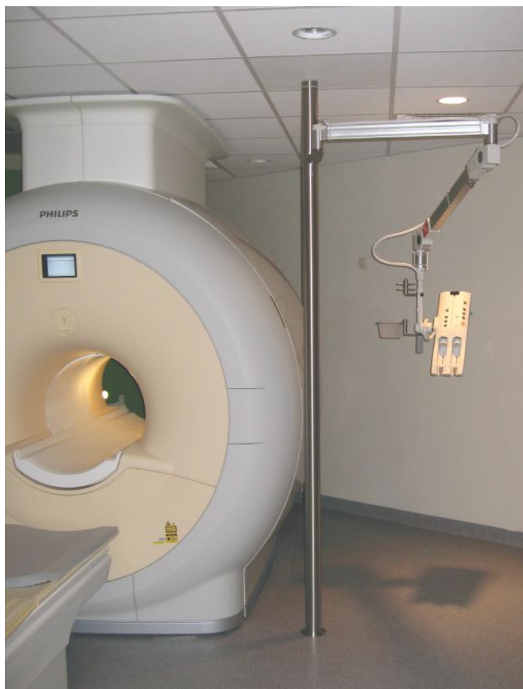
Above: Pole mount installed tight to MR Gantry Left: Plywood cemented to Faraday RF Shield provides ceiling fastening without shield interference. Patent Pending
