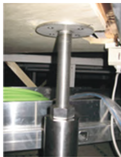
Above: Pole mount installed tight to MR Gantry Left: Plywood cemented to Faraday RF Shield provides ceiling fastening without shield interference
