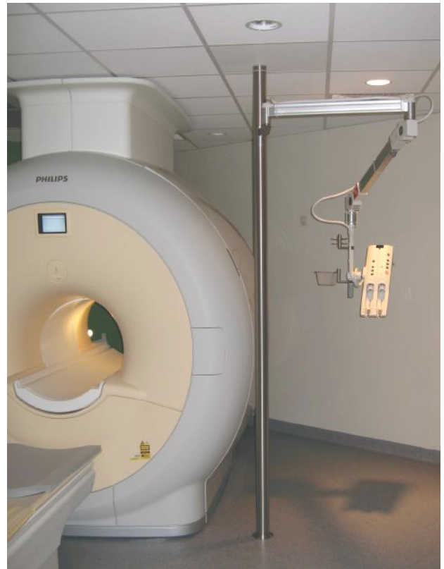
Above: Pole mount installed tight to MR Gantry Left: Plywood cemented to Faraday RF Shield provides ceiling fastening without shield interference
