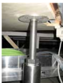
Above: Pole mount installed tight to MR Gantry Left: Plywood cemented to Faraday RF Shield provides ceiling fastening without shield interference. Patent Pending
